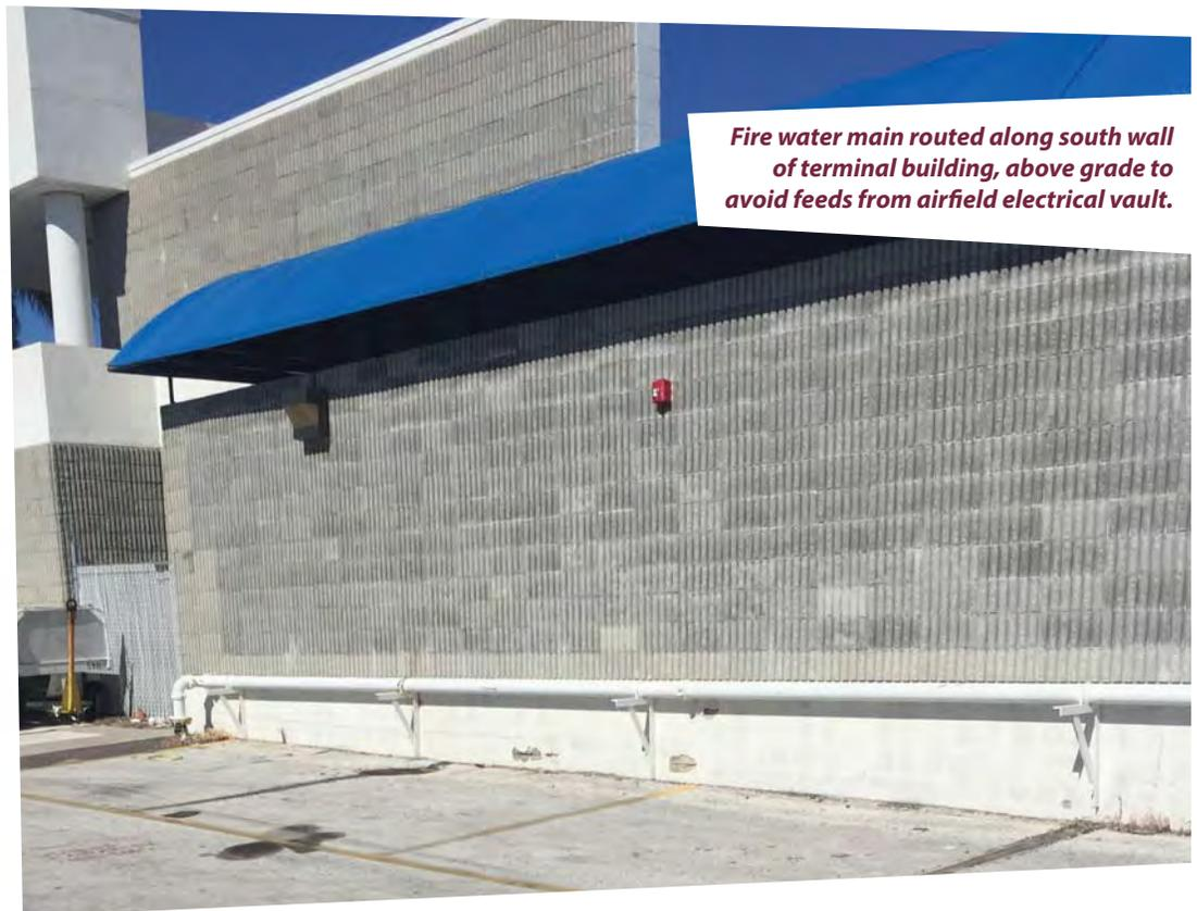
*Fire water main routed along south wall of terminal building, above grade to avoid feeds from airfield electrical vault.*
