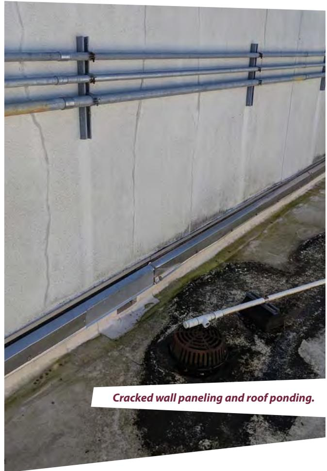
**Cracked wall paneling and roof ponding.**
