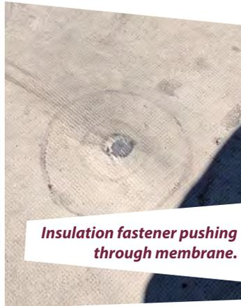
**Insulation fastener pushing through membrane.**
