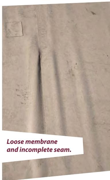
**Loose membrane and incomplete seam.**
