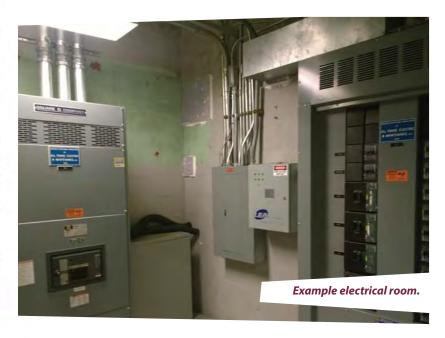
The main distribution boards feeding the electrical rooms and panels throughout the airport range in size from 800 amps to 4000 amps depending on the size of the area it is serving. From these distribution points the main feeders to the various areas of the airport are either individually metered via a combined meter center to allow
