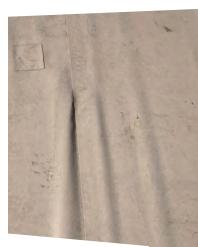
Loose membrane and incomplete seam.
