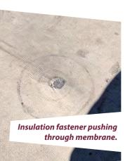
that are starting to push on the membrane, and in some instances have punctured the membrane.
